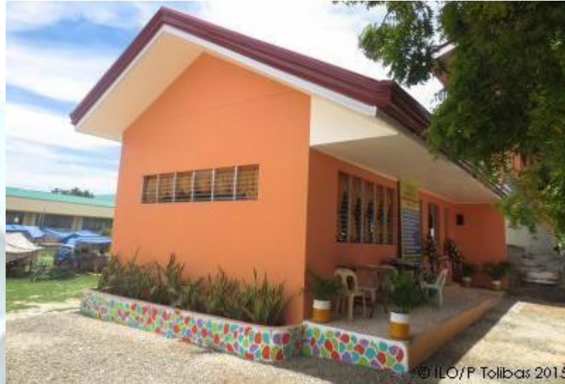
Figure 7: Exterior view of the Livelihood Center
